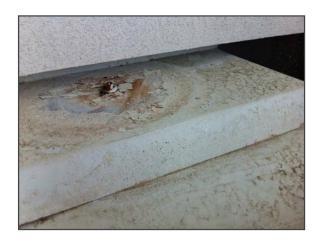
Another example of roof damage due to a overhanging roof design, note the dirt build up in this sheltered area which natural rainfall doesn't reach and which cannot be routinely rinsed down due to it's inaccessible location.
