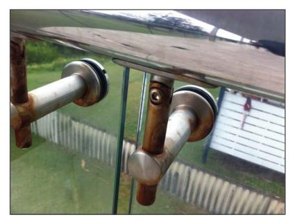
This balcony has highly polished handrail and satin finish supports. The handrail is unaffected, however, the satin finish supports have corrosion even though they are the same grade of 304. We used Action Rust Removal Cream, a gentle safe cream formula to restore the supports and Action Clear Coat to protect it from future corrosion.
