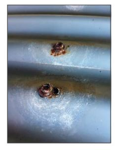
This Pavilion design with roof overhang, prevents rain water washing down screw heads, allowing salt to settle and rust to take hold. Remember rain runs down the valleys of the roofing, leaving the screws generally untouched. This roof is five years old and the screws are too rusted to be removed. You can see rust appearing in the sheet surrounding the screw head. Whilst the metal roofing has a warranty, it does not extend to damage as a result of screw heads.
