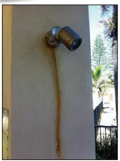
This is the usual outcome when poor quality hardware is used to affix lights and other fittings to a masonry wall. In this instance remove fitting, replace screws with stainless steel and coat with Action Clear Coat. To remove rust staining from wall use Action Gel as shown below.
