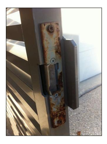
Keep metals which are in contact the same wherever possible. If this is not possible, ensure that they can co-exist by referring to the Galvanic Corrosion Tables (following page). The zinc plated striker plate in this picture didn't stand a chance butted up against aluminium in a coastal environment.
