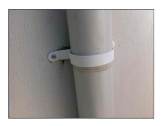
Standard metal down-pipe saddles quickly rust in a coastal location and bleed rust down the walls as shown. We always recommend using plastic or stainless steel saddles wherever possible, as shown right. The plastic saddles can be painted as required.
